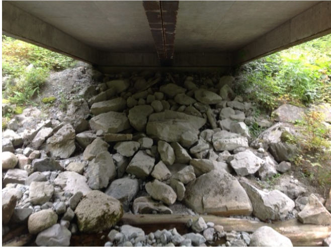
Left Bank Abutment when facing downstream
