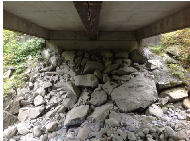
Right Bank Abutment when facing downstream
